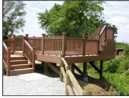
From the deck, visitors will be able to look into the remnant cut and enjoy the fantastic view to the north and northwest. The structure is treated lumber with the decking built with a product call Timber Tech, a recycled plastic/wood composite that allows us to meet our mission of using recycled products, not to mention that it provides fantastic durability and low maintenance."
