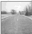
In the 1930s, for some unknown reason, this section of Route 66 was resurfaced. The original Portland cement was covered with brick, and the grade widened to a width of 20 feet [left].
