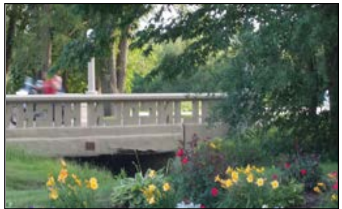
The Lincoln Highway Bridge and Friendship Garden in Tama.
