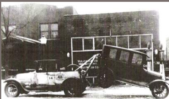
Sankot Garage self-made wrecker made from a 1929 Cadillac chassis.
