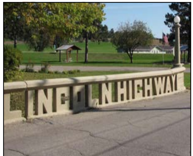
The Lincoln Highway Bridge in Tama.
