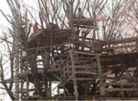
Early spring when most of the work was completed.
